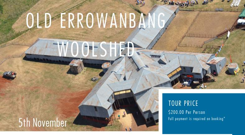
Old Errowanbang Woolshed is a heritage-listed shearing shed at Errowan Park, Old Errowanbang Lane, Errowanbang, It was designed by Watt and built in 1886. The shed is unique in that it is constructed on four levels, all of which can be operated separately depending on demand. From the exterior these levels are clearly seen as distinct wings radiating from a central control room. The large complex has 40 shearing stands, of which 26 have never been adapted for mechanical shearing.
